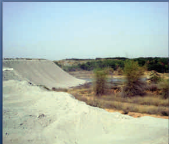
The ash dump of a coal plant in Orissa. Note the location of the dump on the banks of a water body
